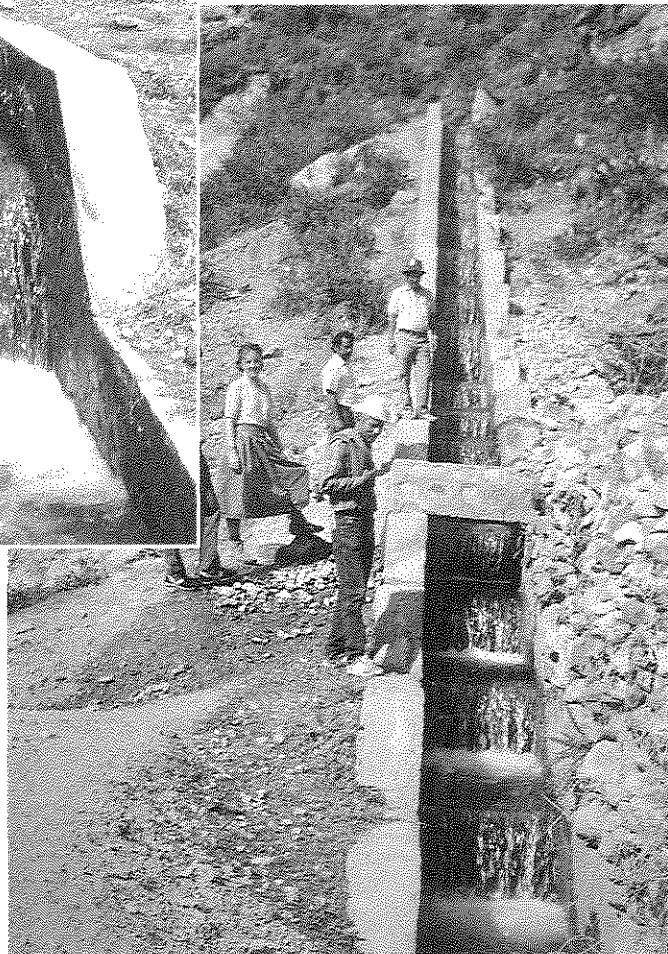
Photograph 5B A Cascade Drop Structure in Stone Masonry
