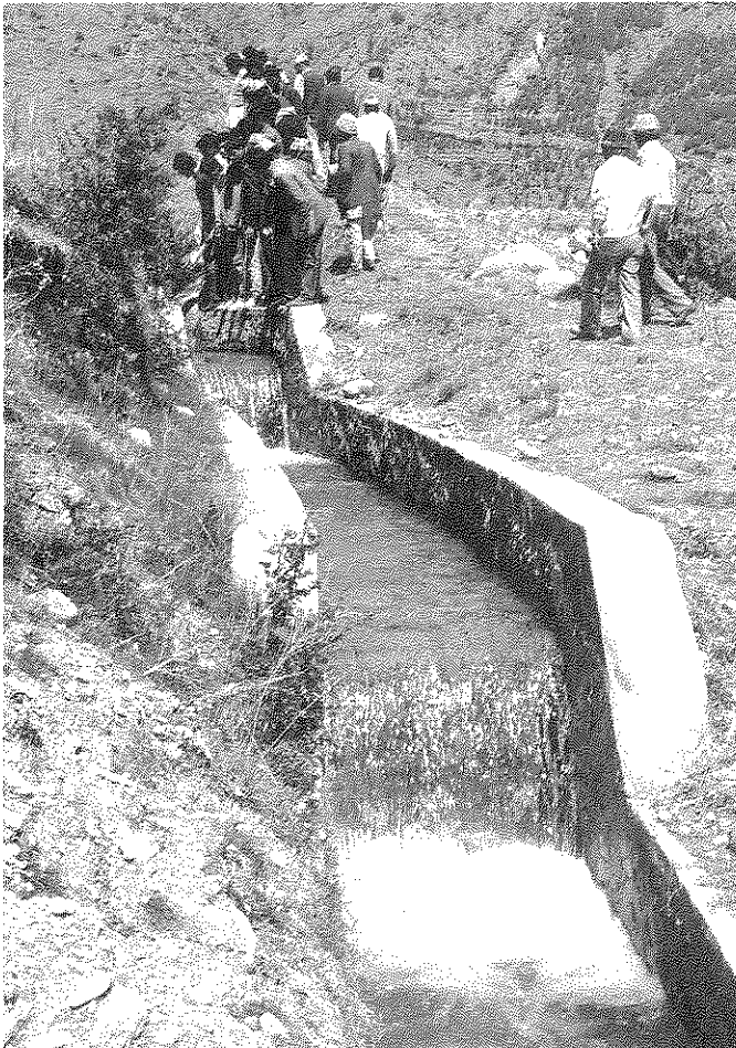
Photograph 5A A Vertical Drop Structure in a Masonry Lined Canal
