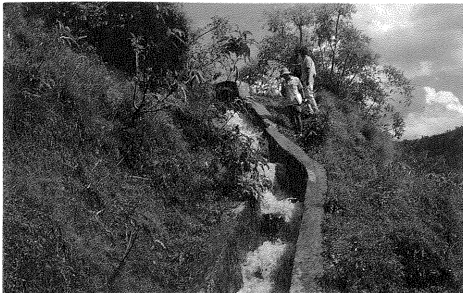
Photograph 5C A Cascade Drop Built in Strong Masonry
