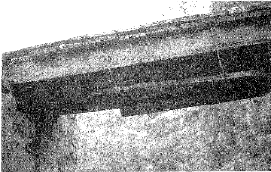
Photograph 4J HDP Pipe Aqueduct Supported With Timber Beams
