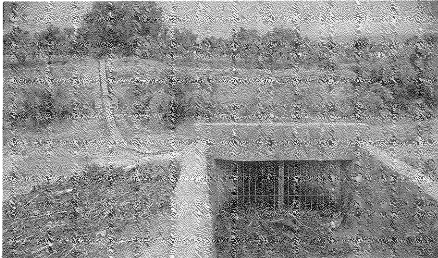
Photograph 4C Shallow Siphon in Reinforced Concrete
