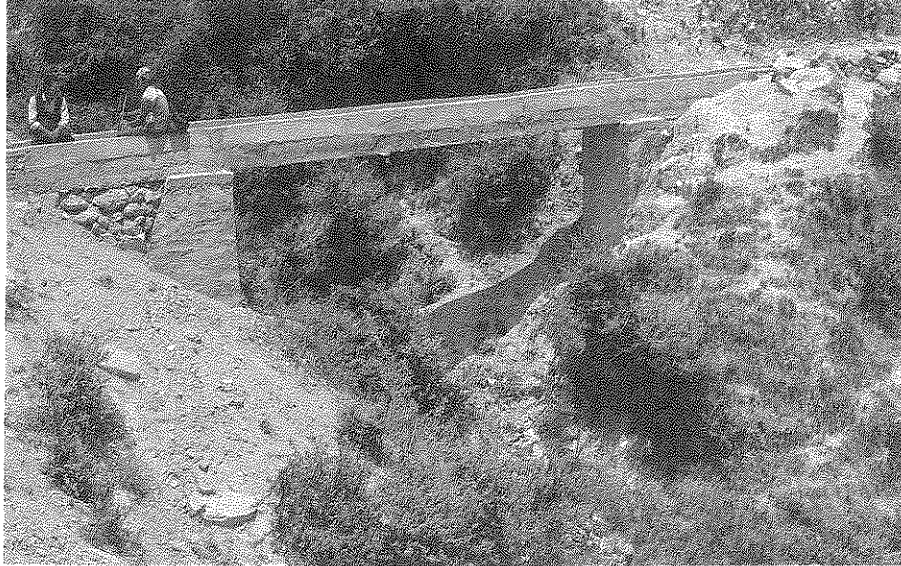
Photograph 4F Reinforced Concrete Single Span Aqueduct Supported on Masonry Abutments
