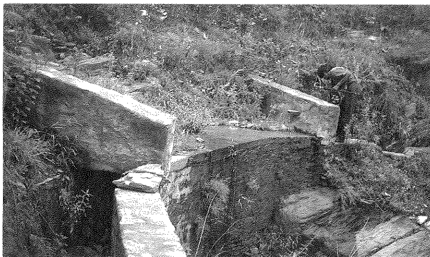
Photograph 4B Super Passage Over a Masonry Lined Canal
