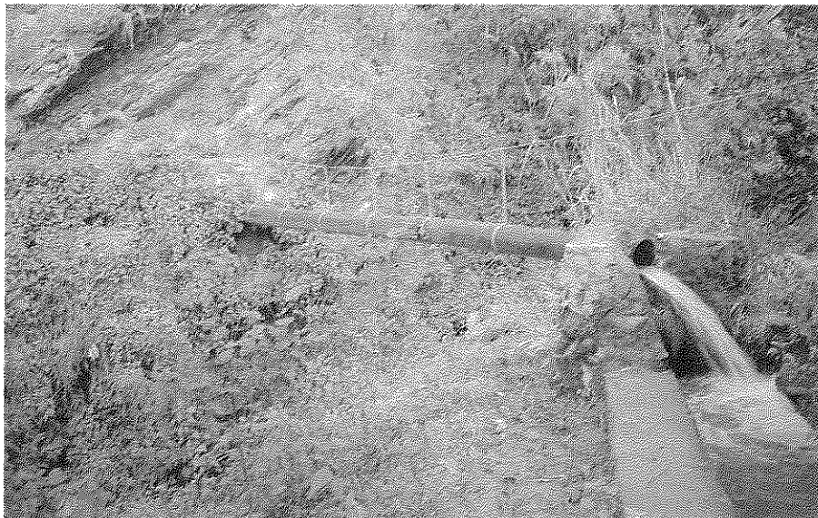
Photograph 4G Suspended Polythene Pipe Aqueduct: Span approximately 7 metres
