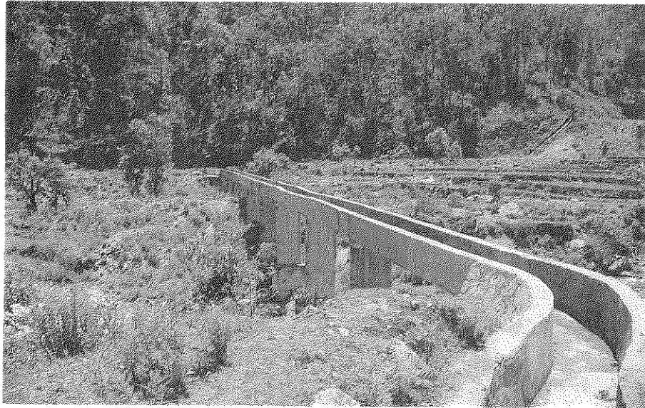
Photograph 4H Reinforced Concrete Multi-Span Aqueduct
