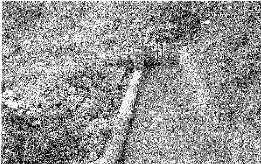
Photograph 2C Settling Basin with a Long Fixed Crest Side Spill
